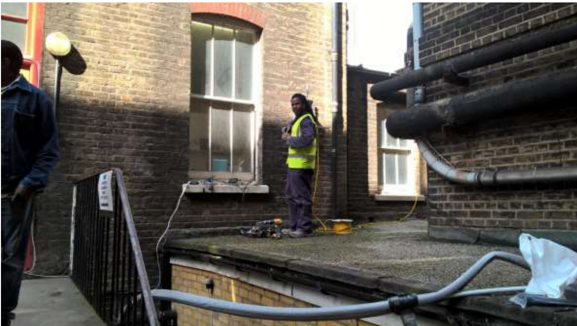
Figure 6 Middlesex Hospital Annex 2 (Behind Electrician)
